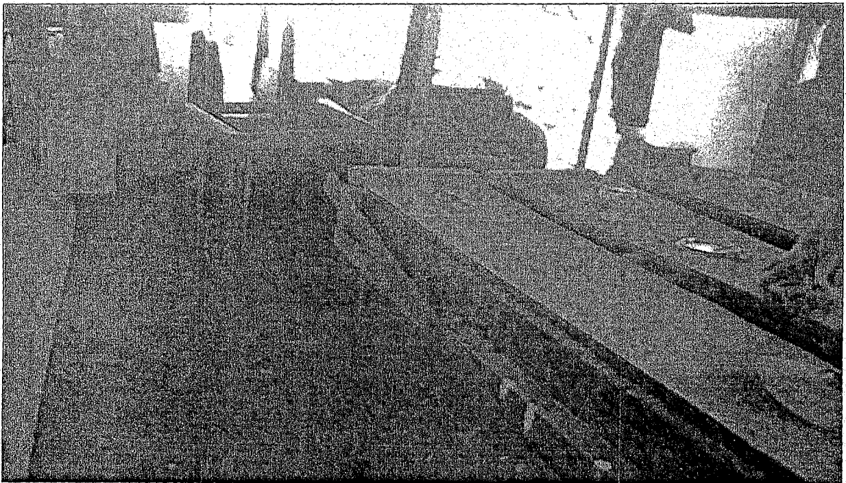
PLATE 17: SHOWING THE INTERIOR SPACE OF A SHOP IN MINNA PARK.
