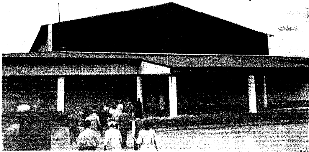
Plate 4a: front elevation of the auditorium in the trade fair complex, Kaduna.
