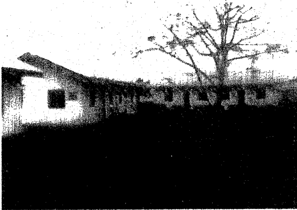
Plate 3.2 View of guest chalets and landscaped area
