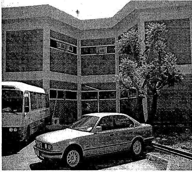
Plate 82 showing part of the offices
