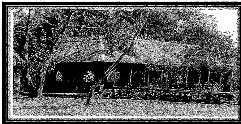
PLATE 3.7: SIDE VIEW OF THE ADMINISTRATIVE BLOCK
