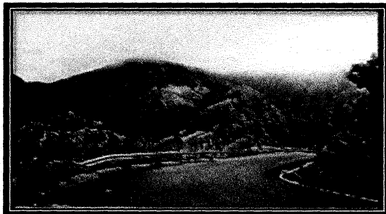
PLATE 3.4: THE ACCESS ROAD TO THE RESORT
