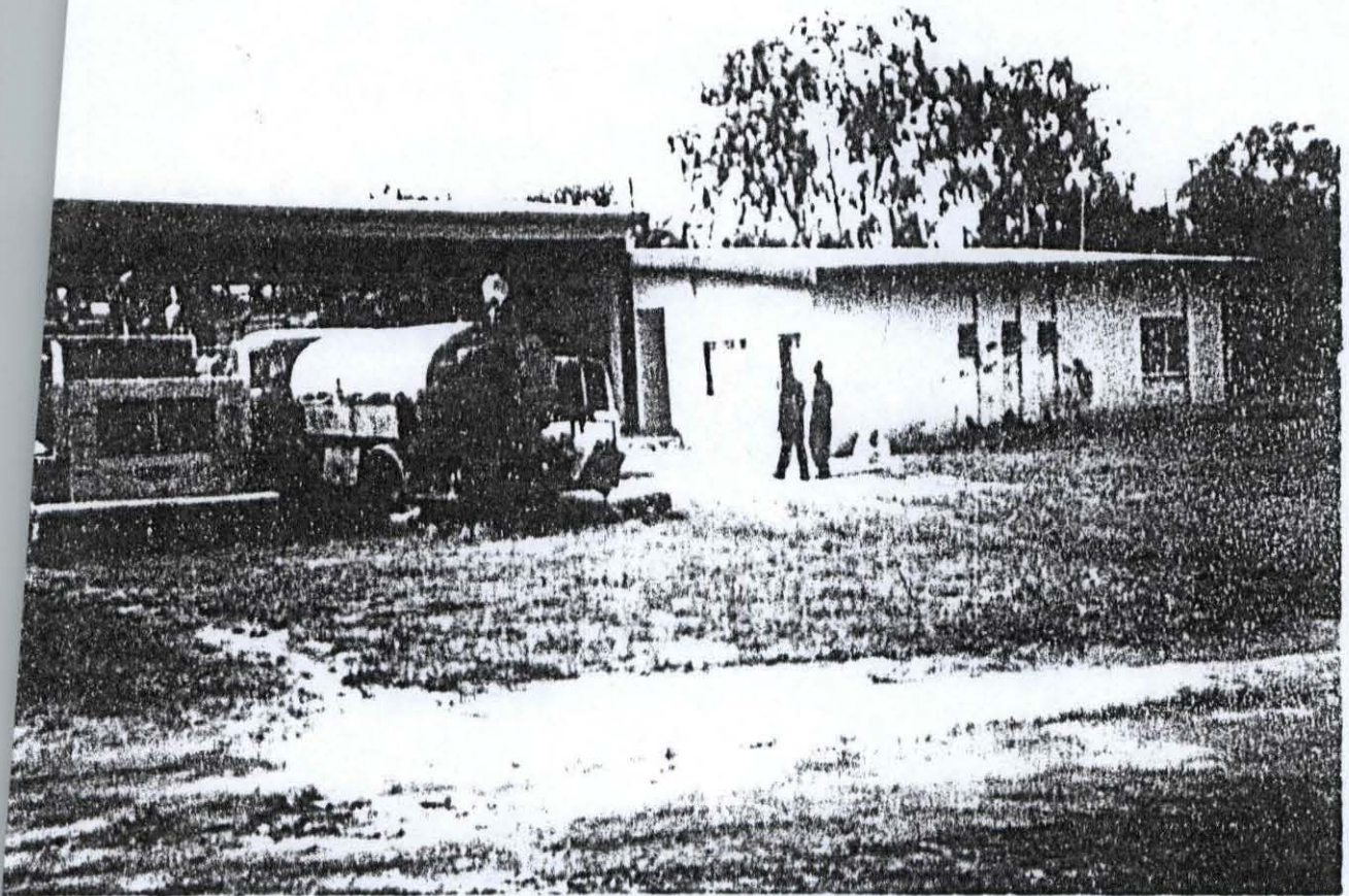
G 4.3.3 SHOWING THE CENTRAL CONTROL ROOM AND MACHINE BAY REAR VIEW
