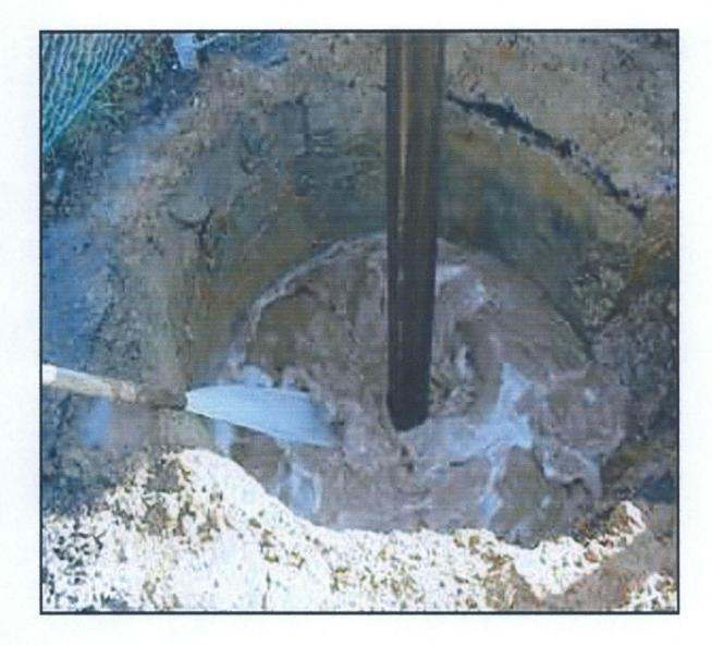
Figure 2.3: A typical Drilling Mud
