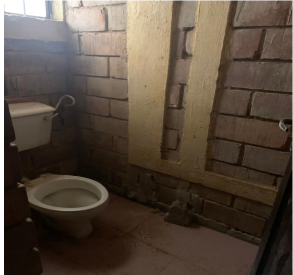
Figure 4.7 Gidan kwano Female Hostel Toilet
