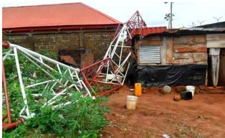
Plate I: Lagos tower collapse (Source: Akoni, 2014)
