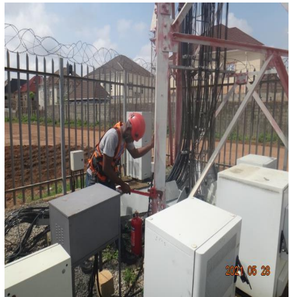
Plate XIX: Bolt torquing
