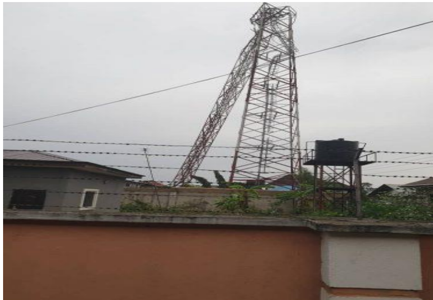
Plate V: Akwa Ibom tower collapse I (Source: Tom, 2021)
