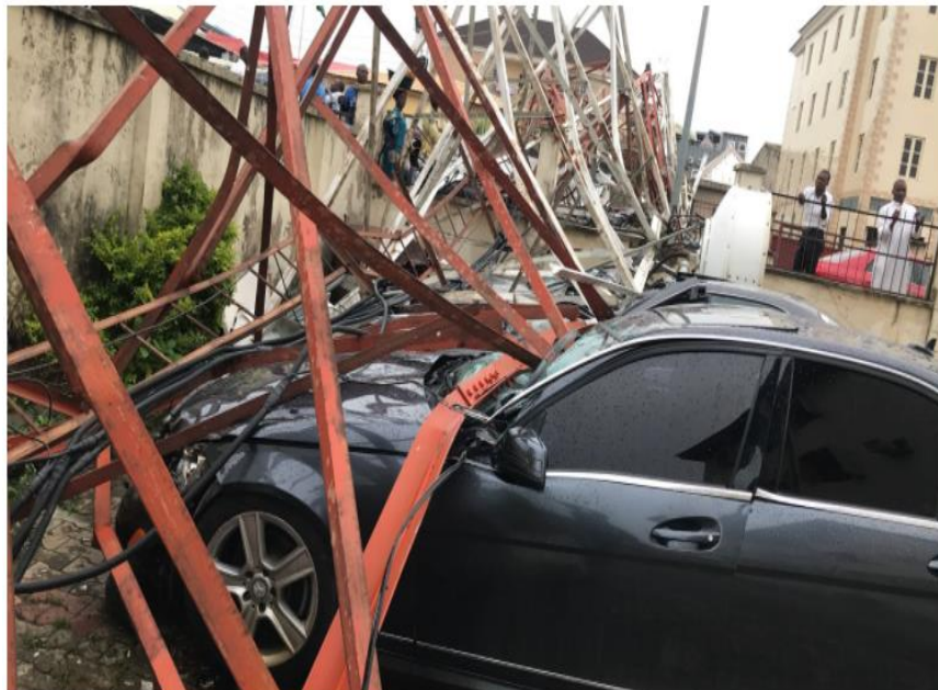
Plate III: FCT tower collapse ( Source: Ikeji, 2019)
