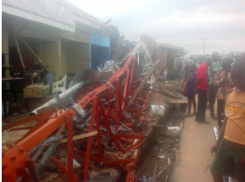
Plate II: Cross River tower collapse ( Source: Kalu, 2014)
