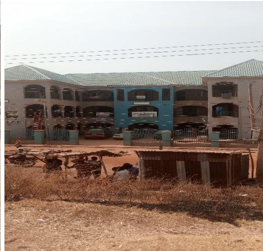
PLATES II: A two storey complex at Barikin Sale
