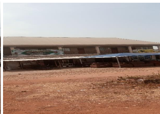
PLATES VI: A single storey complex at Western Bypass
