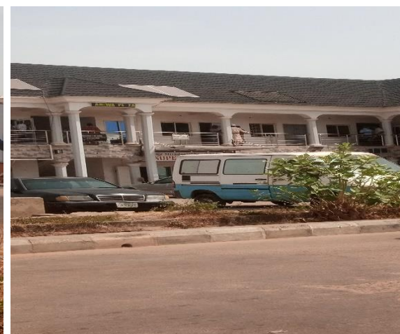
PLATES XII: A Two storey complex at Shiroro road
