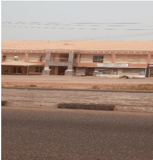
PLATES VII: A single storey complex at at Western Bypass
