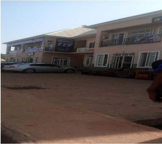
PLATES XV: A two storey complex Shiroro road
