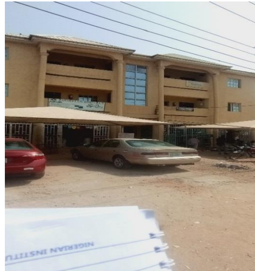
PLATES VIII: A Two storey complex Paiko road
