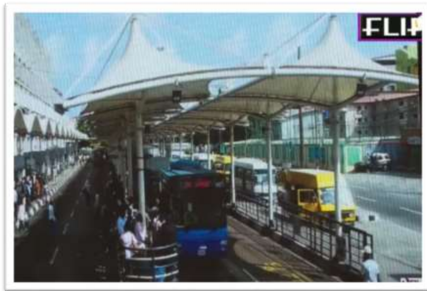
Figure 4.14: Ikeja terminal cover loading bay.
