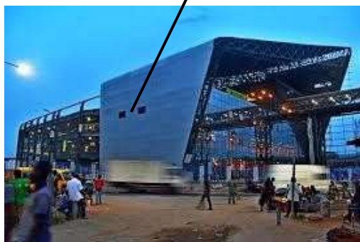
Figure 4.6: Oshodi terminal building Source: Autoreporting.com, (2020)
