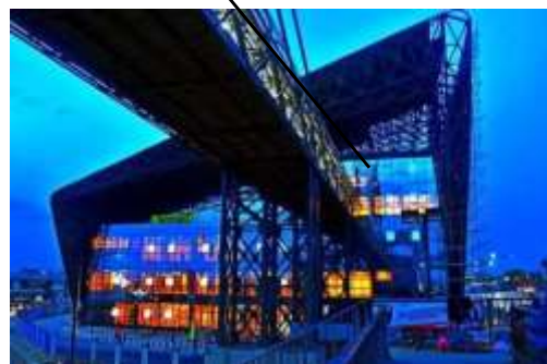
Figure 4.7: Oshodi pedestrian overpass Source: Autoreporting.com, (2020)
