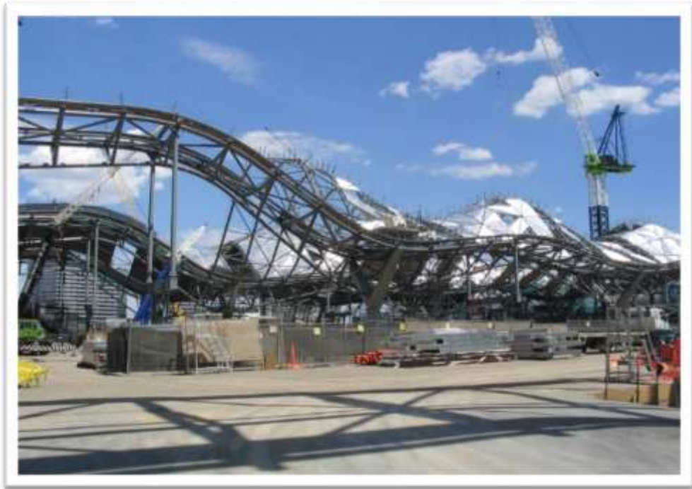
Figure 4.31: Melbourne roofing structure of the new spenser street. Source: Skyscanner, (2020).
