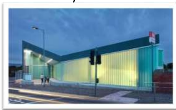
Figure 4.24: Dalmanock station platform Source: Achidaily.com, (2020)
