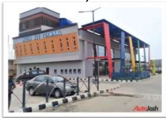
Figure 4.10: Ikeja terminal building Source: Nairaland, (2020)
