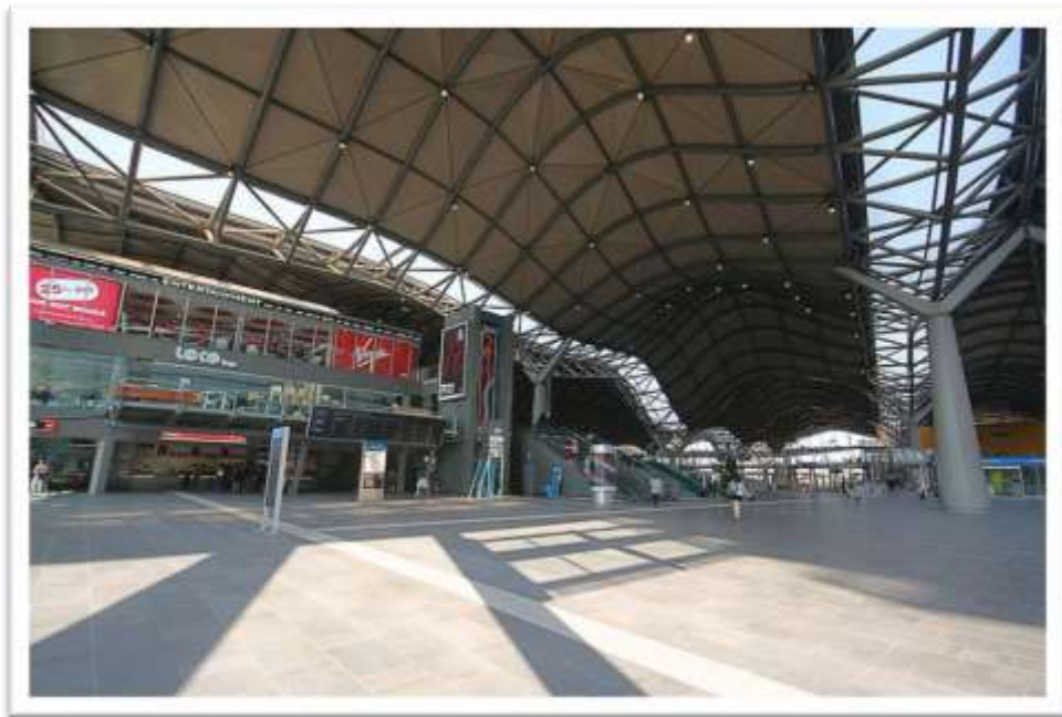
Figure 4.32: Melbourne passengers waiting area. Source: Skyscanner, (2020).
