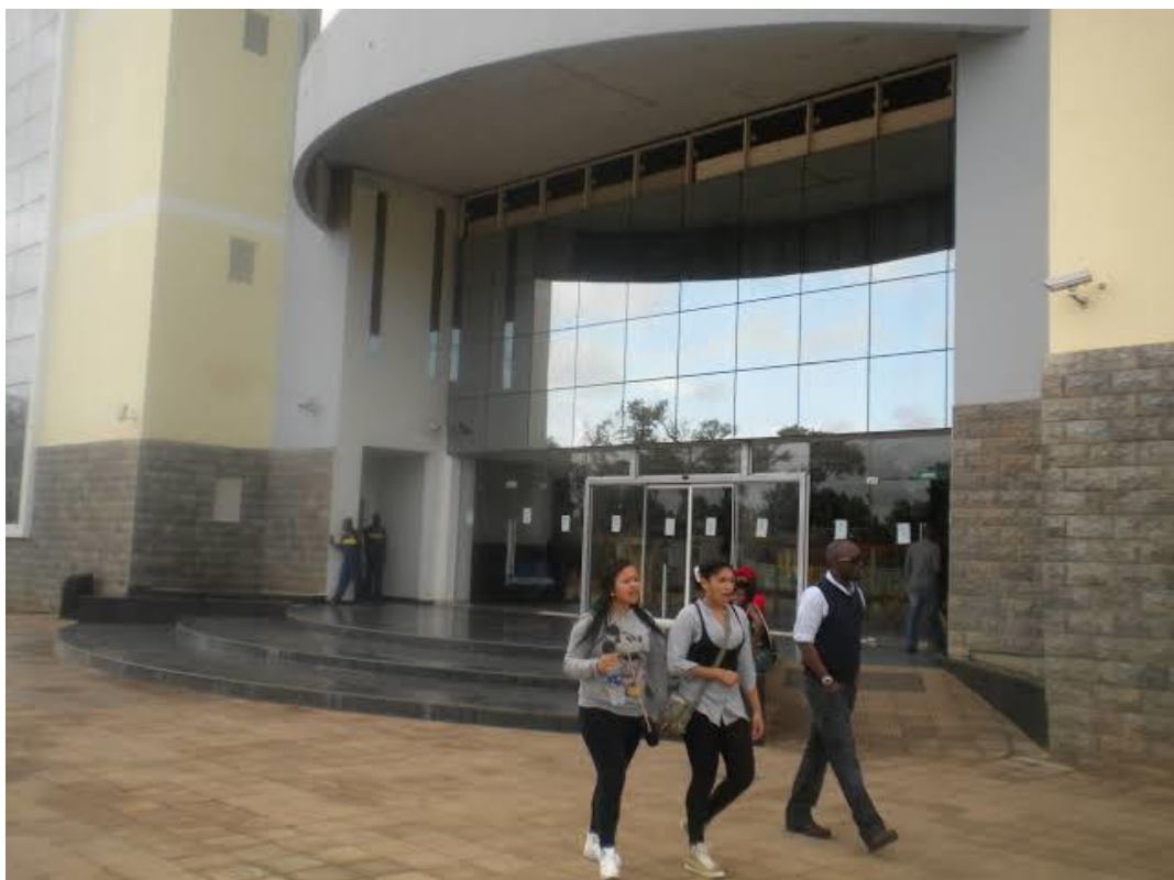
Plate XII: Pedestrian walkways, Silverbird Galleria, Abuja Source: Author's fieldwork (2020)
