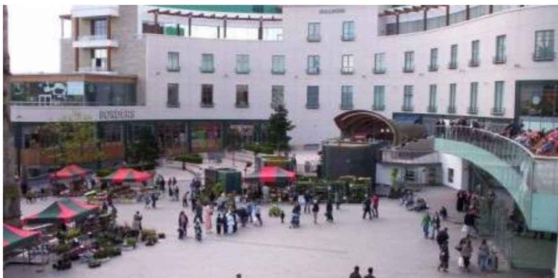
Plate XXXIV: Windows, Bullring, Birmingham Source: Author`s fieldwork (2020)
