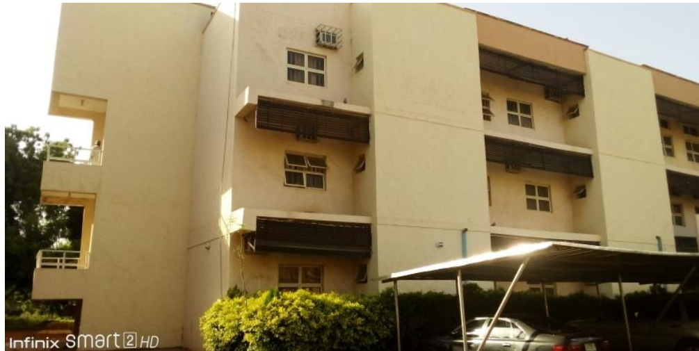
Plate V: Roof Overhang at UDUS Source: (Author's fieldwork, 2019)
