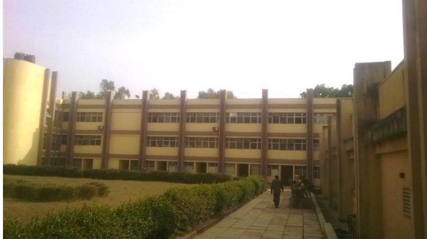
Plate IV: Shading devices at ABU Source: (Author's fieldwork, 2019)
