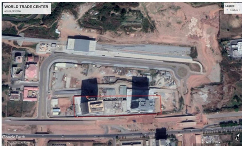
Plate IV: Aerial view of site of the world trade centre Abuja
