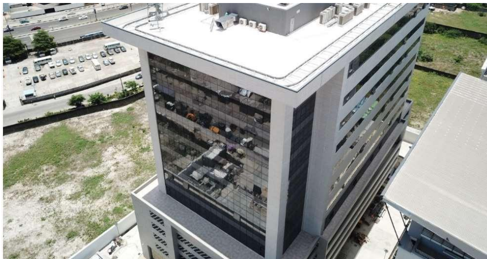
Plate VIII: Insulated roof and higher thermal performance glass during daylight
