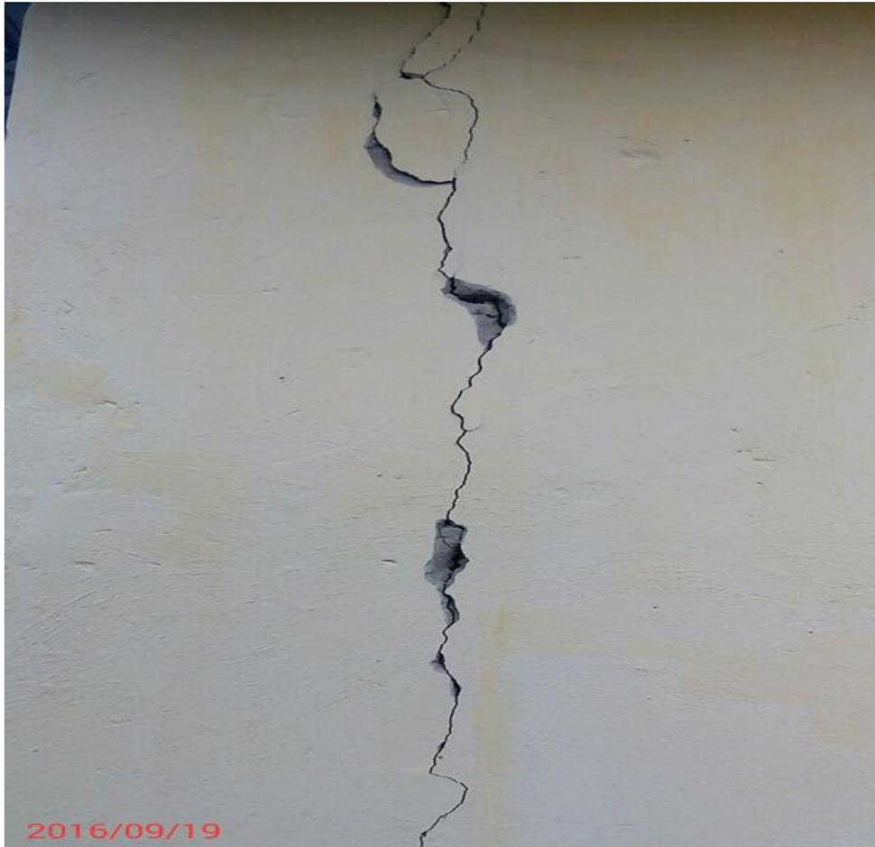
Plate II: Affected structures in Kwoi town, Nigeria, as a result of the 2016 earth tremor
