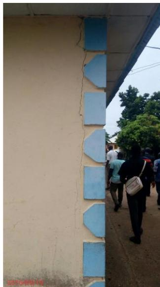
Plate VII: Crack on a newly constructed building in Kwoi Town
