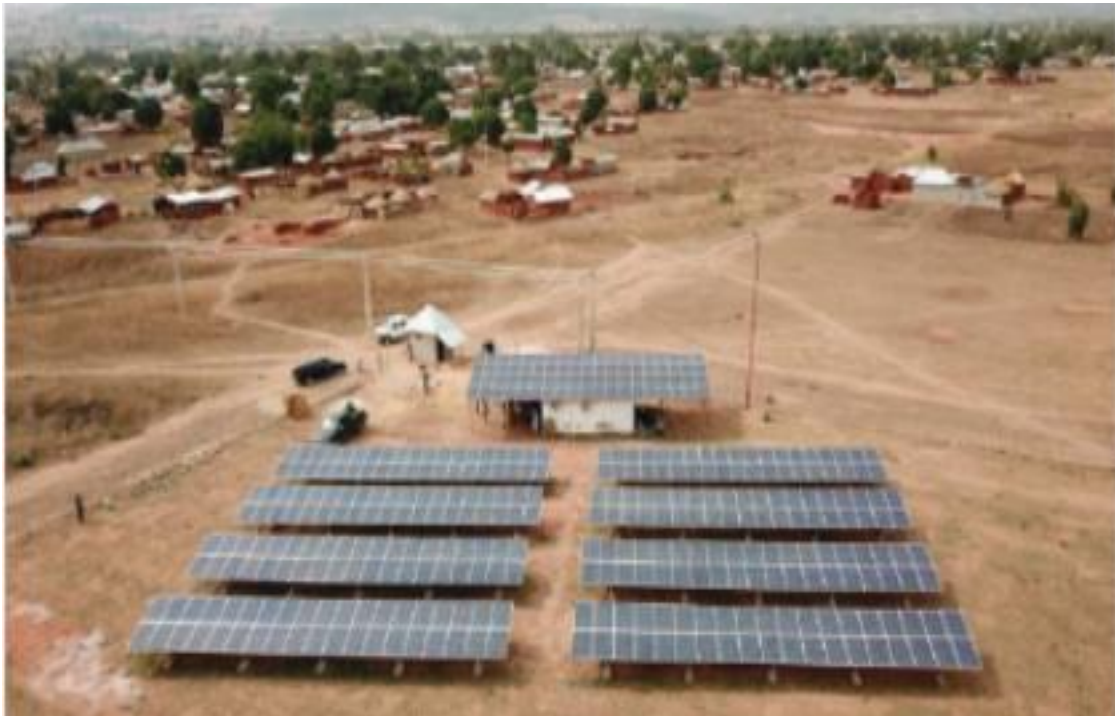
Plate 2.1: Tungan Jika solar mini-grid
