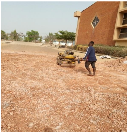
Plate VI: Compaction with light roller Plate VII: Compacted finished surface.
