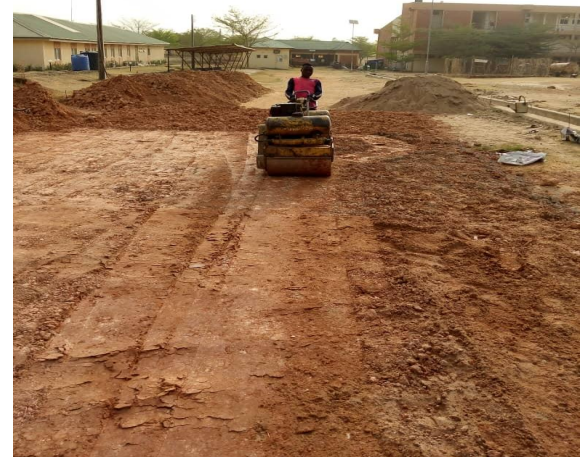
Plate V: Compaction with light roller
