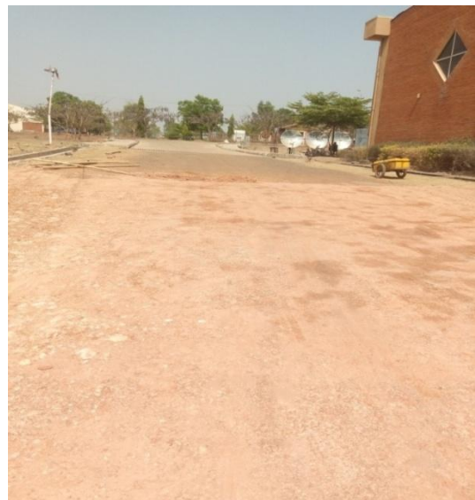
Plate VI: Compaction with light roller Plate VII: Compacted finished surface.
