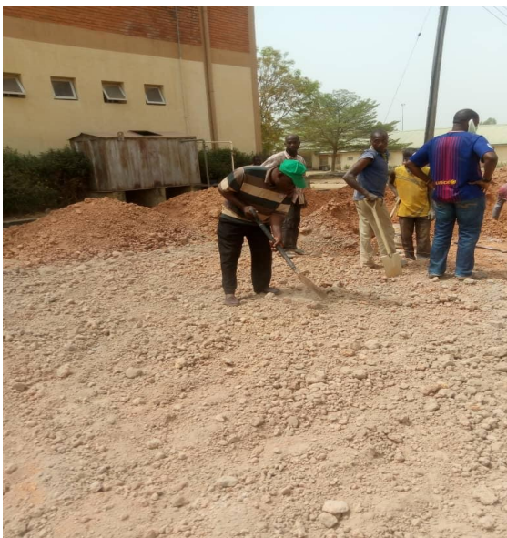
Plate IV: Dry mix of soil, cement and CCR.
