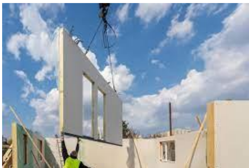
Figure 1: Assembly Process of Prefab Element
