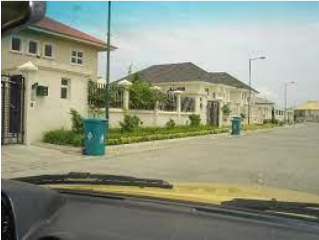
Figure 3: Buildings in VGC, Lekki, Lagos accessed online 09/05/2022
