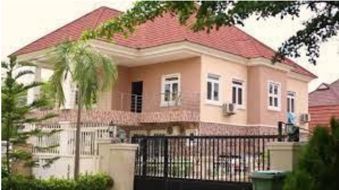
Figure 10: A storey Building Erected with the Stay-in-Place Form Construction by CITEC
