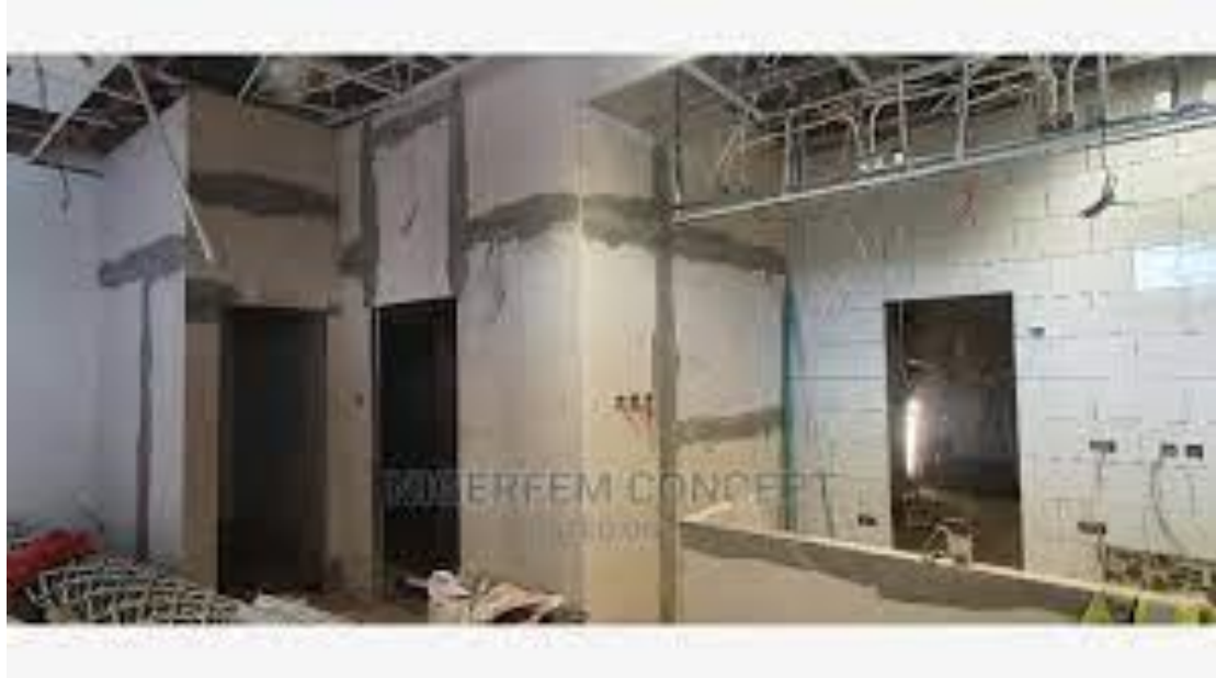
Figure 6: GFRG Panel Construction in Nigeria
