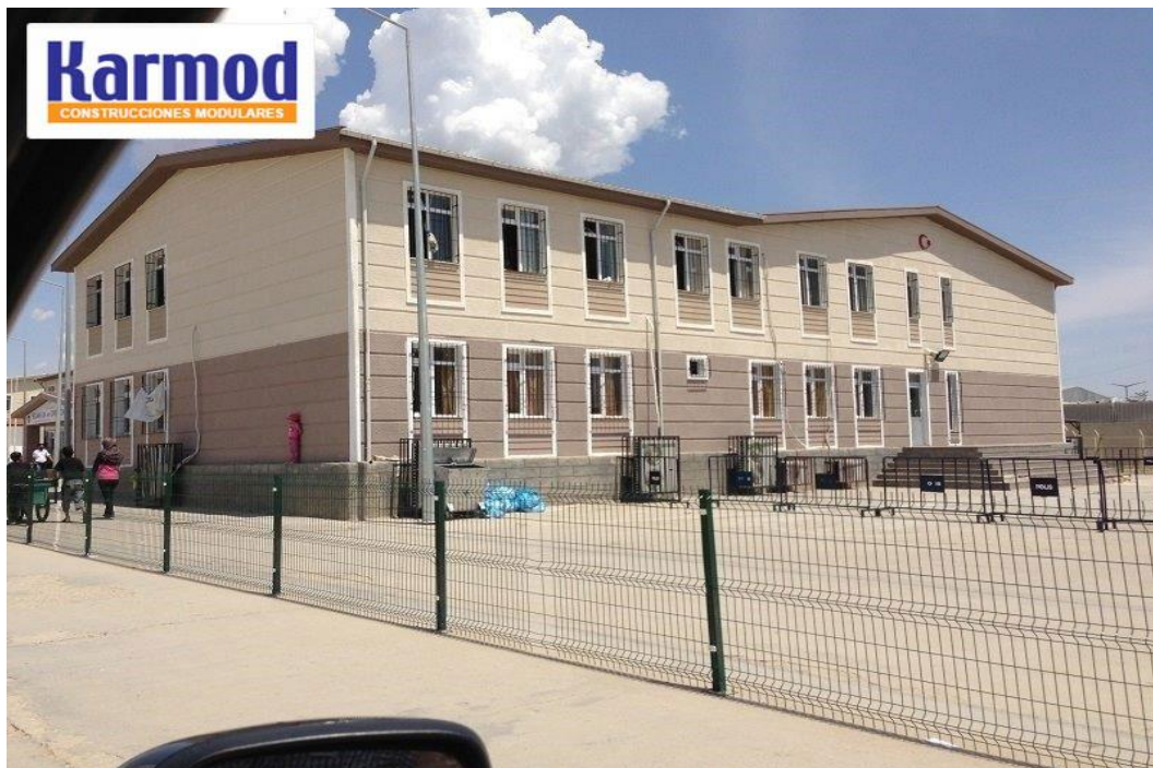
Figure 2:Prefab Building in Nigeria by Karmod accessed online 09/05/2022
