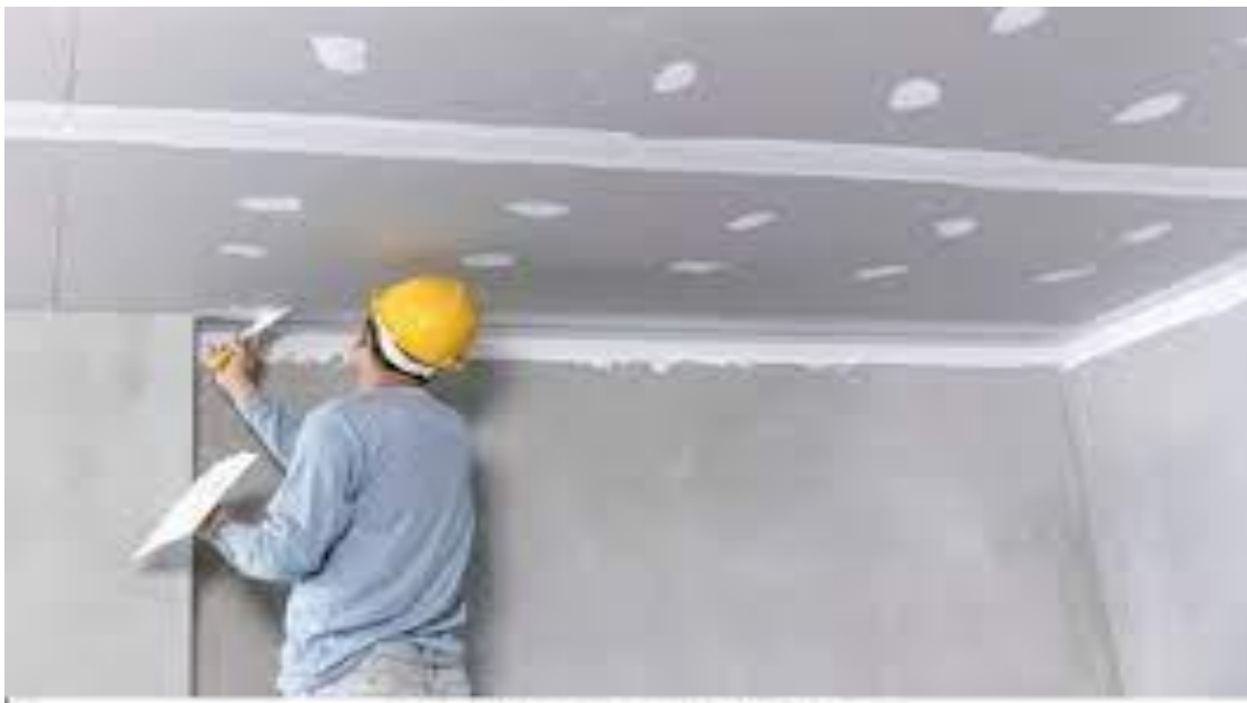
Figure 7: GFRG Panels Construction accessed online on 09/05/2022
