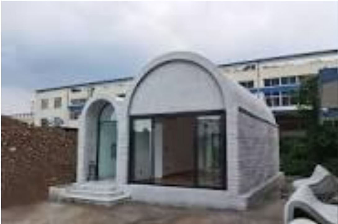
Figure 14: 3D Concrete Printed Building
