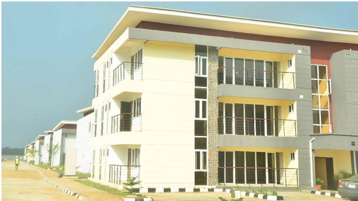
Figure 9: Block of Flats erected with Formwork Construction in Lagos by Alpha Mead Group
