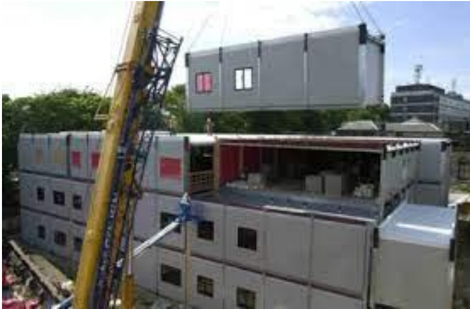
Figure 4: Stacking of 3D Monolithic Modules
