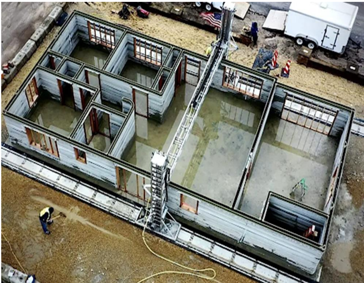
Figure 13: 3D Concrete Printing Arrangement of a Whole Building
