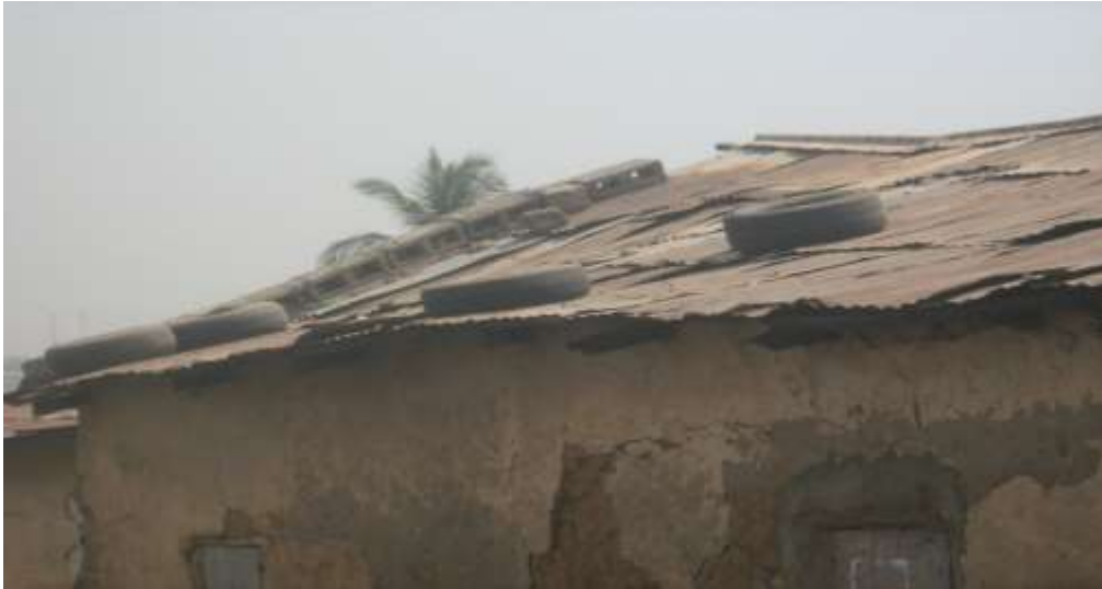
Plate XII: One of the Mitigation Method Adopted in TswataMukun Area Bida Source: Author's Field Survey,2011
