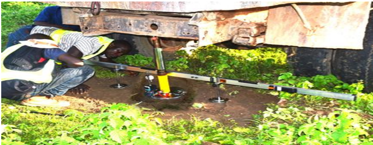
Figure 3. Conventional Plate load test.
