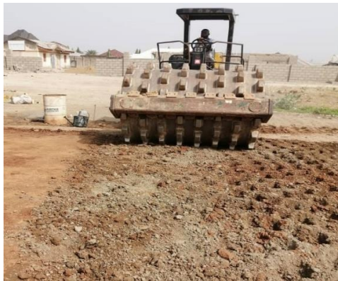
Fig. 4: Compaction of the test sections using sheep-foot roller
