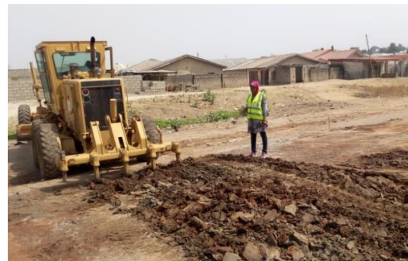
Fig. 2: Scarification of the test sections using ripper
