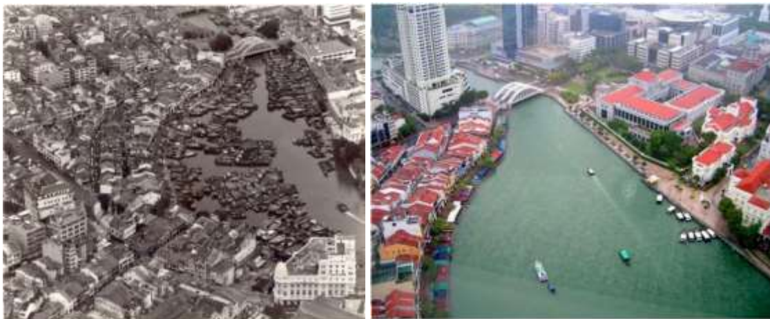
Figure IV and V; Showing picture of Singapore River before and after development of waterfront design approach
