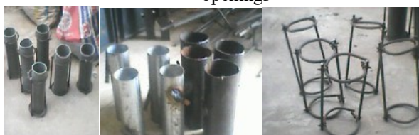
Plate 1: materials used for strengthening the openings
