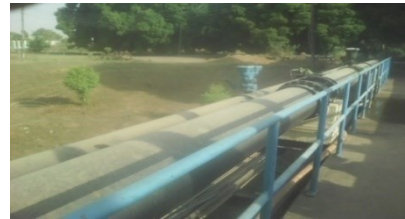
Plate II an asbestos cement pipe
