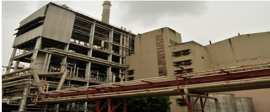
Figure 1: External feature of the power plant (Ajaokuta Steam Power Plant)
