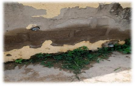
**Figure 2:** Blistering and flaking of mortar within the North Central Region **Source:** www.google.co.uk.images.
