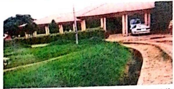
Figure 3: Plate III-Gwamna Awon general hospital Nasarawa road, Kaduna administrative block.
