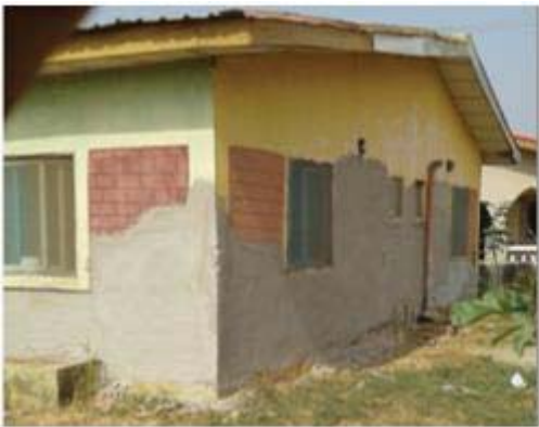
A.1(c): External walls plastered and all roofing sheets replaced
