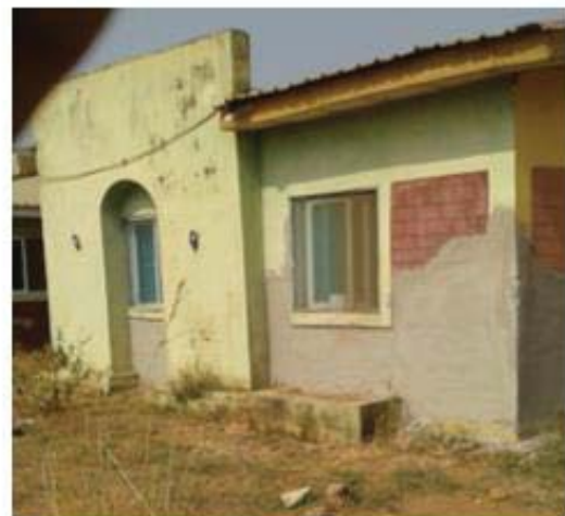
A.1(f): Part of external walls replaced with sandcrete blocks
