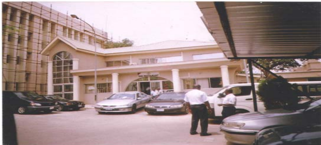
Project 2: Defence Headquarters Officers Restaurant at Area 10, Garki Abuja Source: Authors' Fieldwork, 2015
