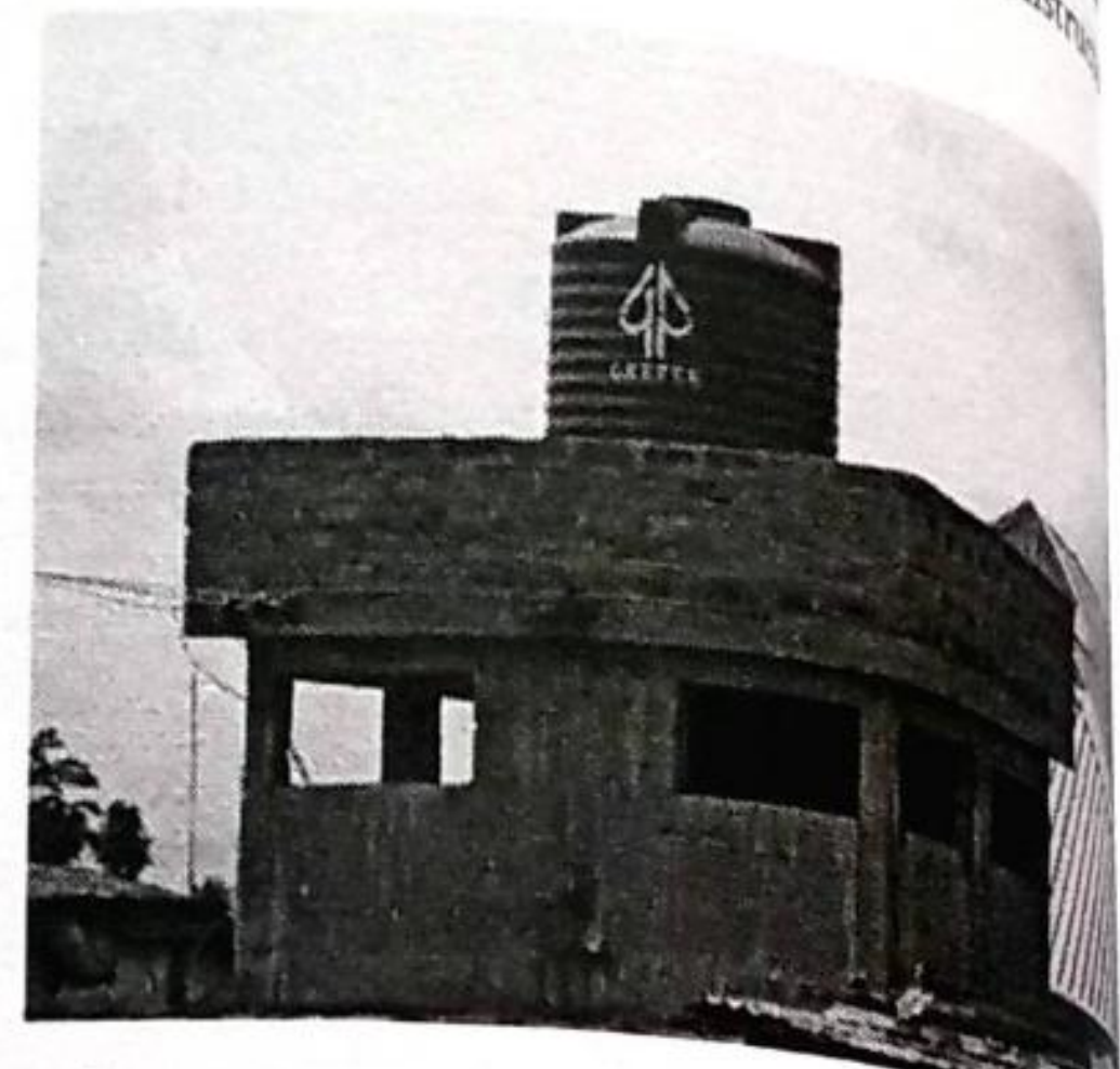
Plate 4: MBB adopted for the perimeter wall of a Water Tank Tower
