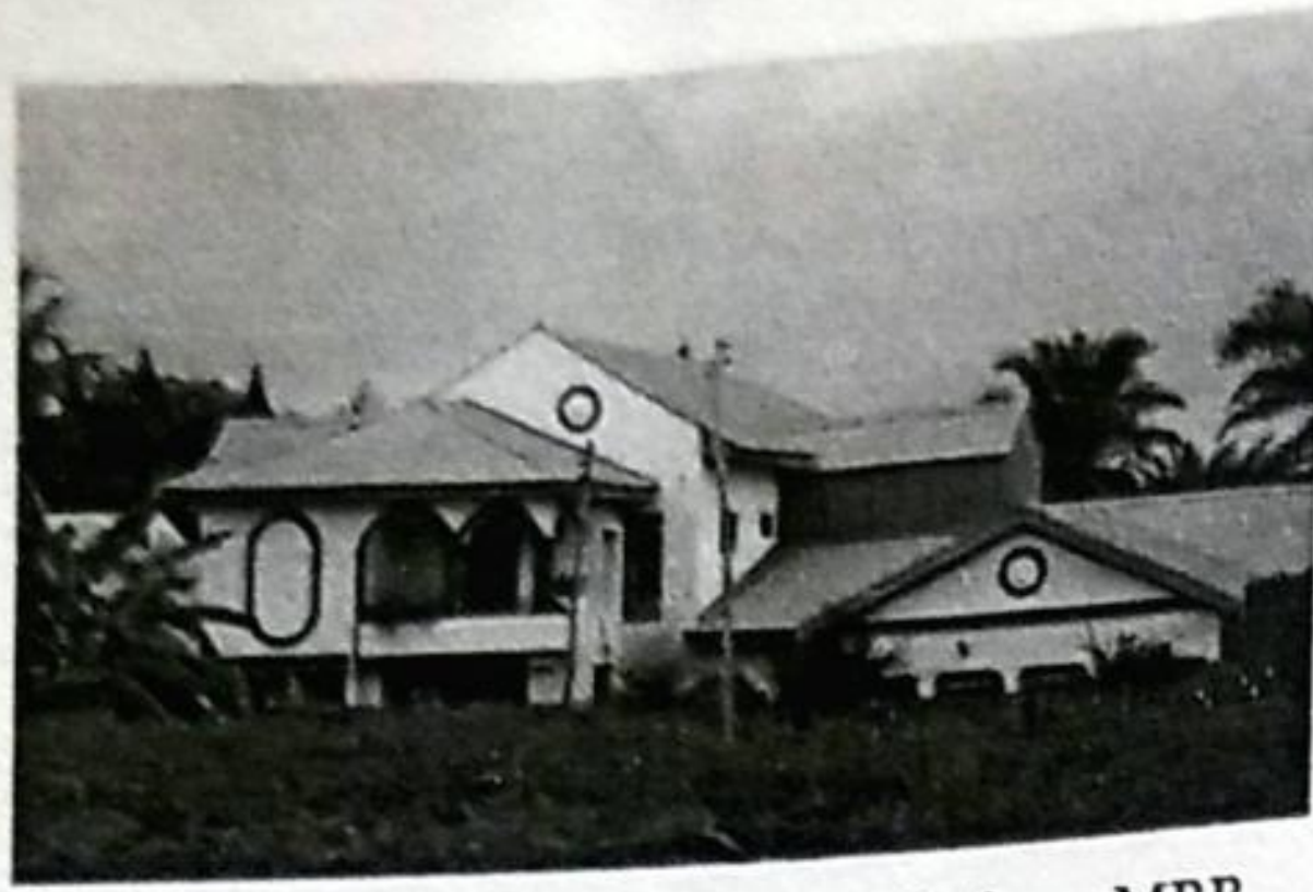
Plate 1: A modern structure built from MBB
