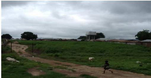
Overhead Water Tank and Telecommunication Mask
