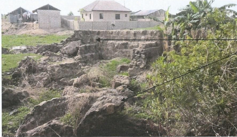
Plate 1: Failure of remedial measure on River Yashi
