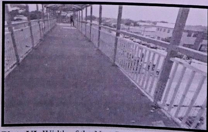
Plate VI: Width of the New Pedestrian Bridges in Minna
