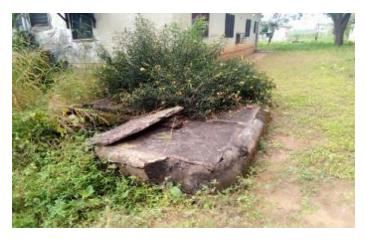
Plate 8: Showing the damaged sock-away
