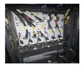
Plate I (a) BTS3900 (An Open Indoor BTS, Vendor: Huawei)
