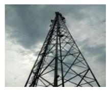
Plate V Tower (For Mounting RF, Microwave Antennas and Terminating Cables)
