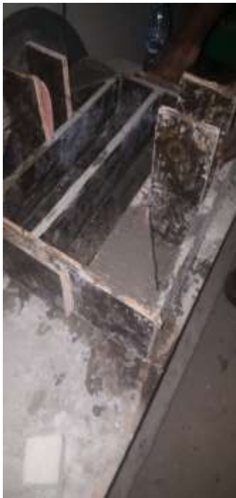
(a) Plain Concrete (Old Concrete) in form
