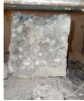
(b) Steel fibre reinforced concrete.
