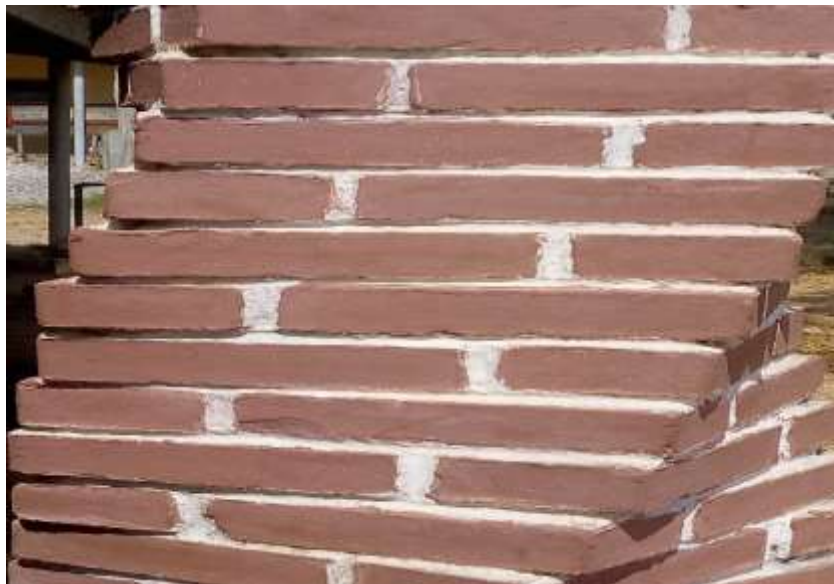
Plate 1: Cement mortar used in masonry work
