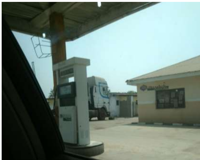
Plate VIII: Light-coloured materials and pitched roof at Bayuk fuelling station
