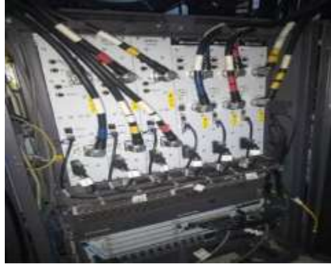
Plate I (a) BTS3900 (An Open Indoor BTS, Vendor: Huawei)
