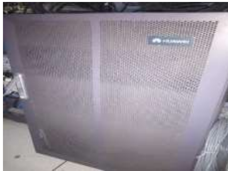
Plate I (b) BTS3900 (Closed Indoor BTS, Vendor: Huawei)
