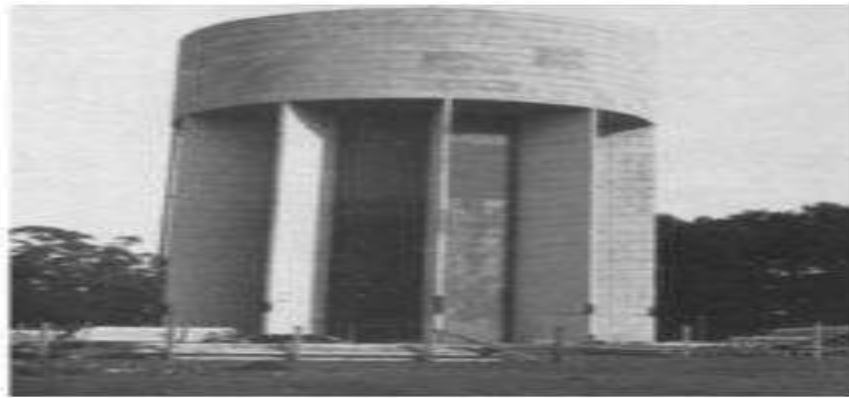
Plate I: Elevated tanks for water supply Source: Muhammad and Safdar, 2020
