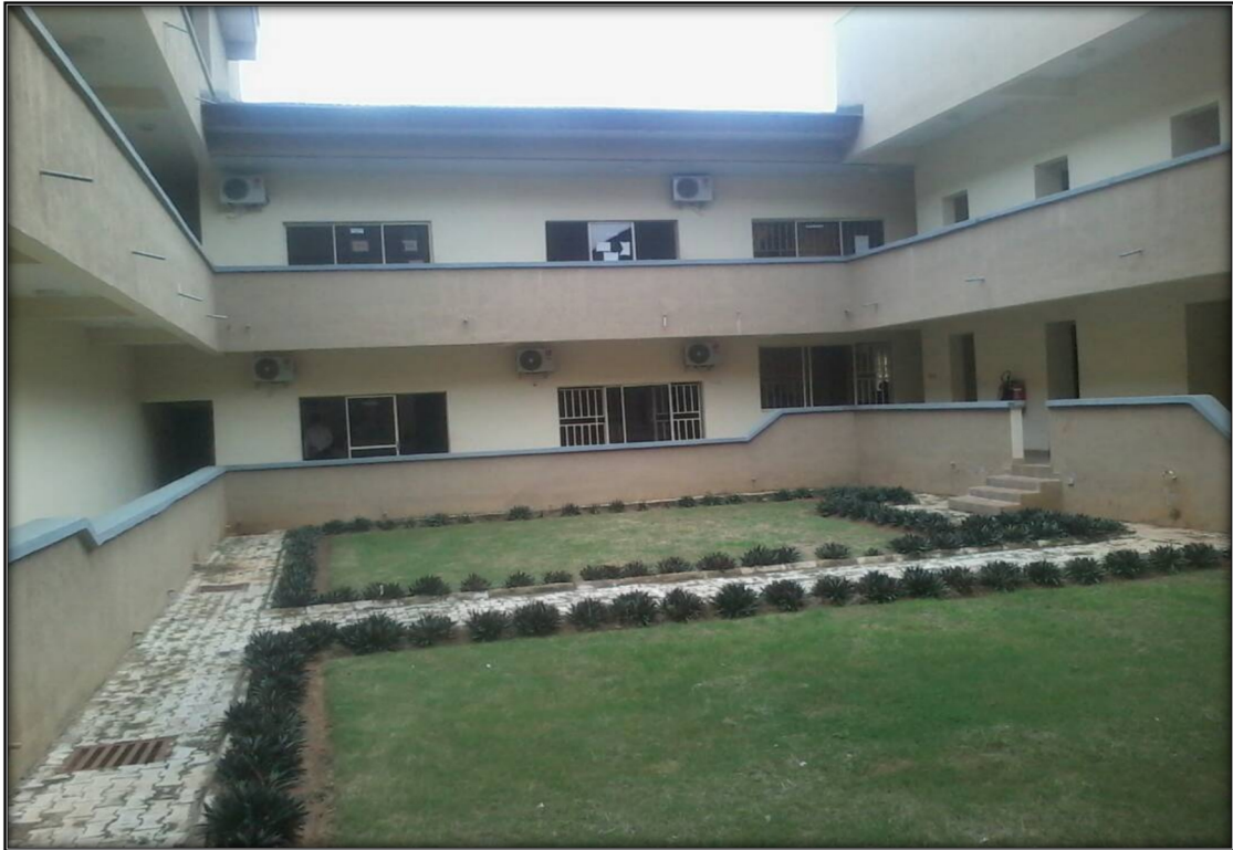
Plate IV: Vertical shading device and large window area in FU Lafia Senate Building (Source: Author's fieldwork, 2019)
