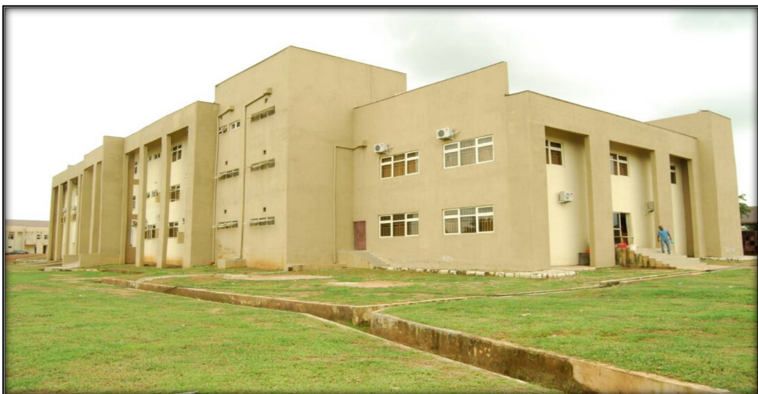
Plate III: Vertical shading device and large window area in FU Lafia Senate Building (Source: Author's fieldwork, 2019)
