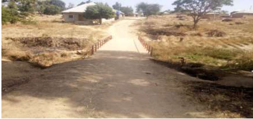
Plate XVII: Exiting Bridge over Stream Channel (Source: Authors Fieldwork, 2018)
