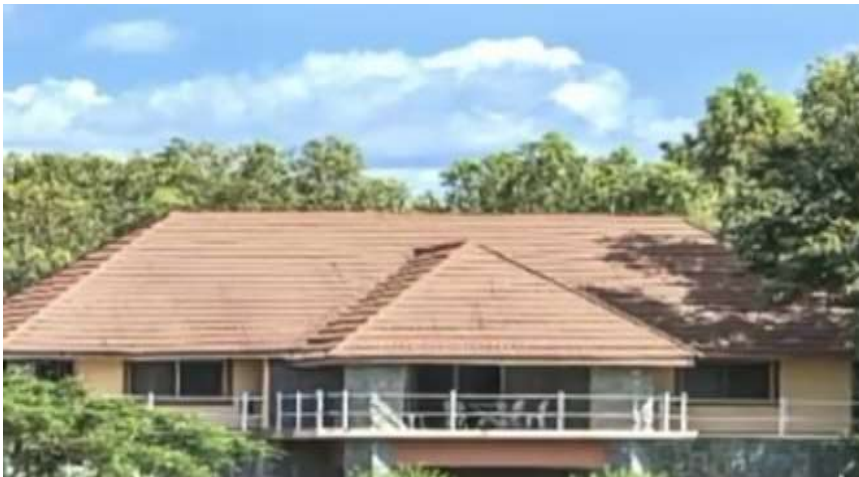
Plate III: A facade view of the polo club house (Source: http://fifthchukker.com 2019)
