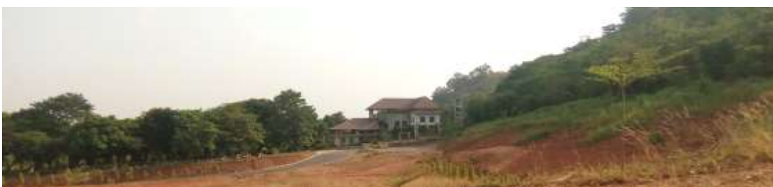
Plate VIII: A view of the polo administrative building (Source: Author's Fieldwork, 2019)
