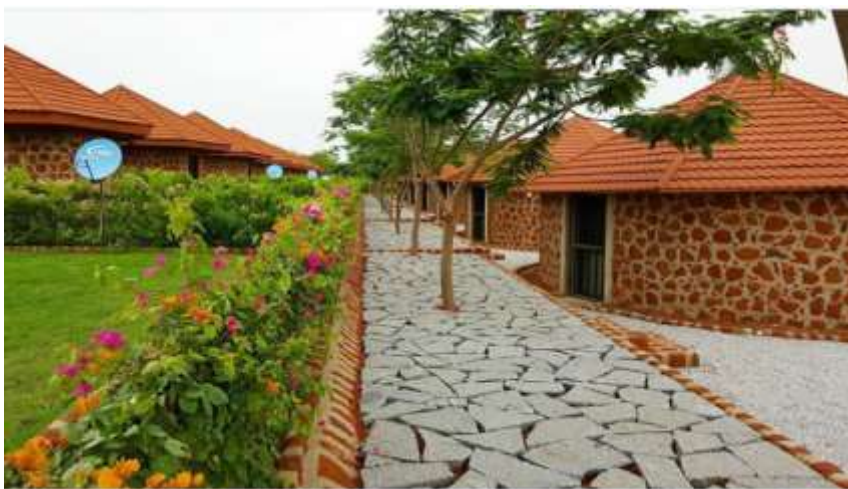
Plate II: A view of the guest chalet. Showing the circular clay huts (Source: Authors Fieldwork, 2019)
