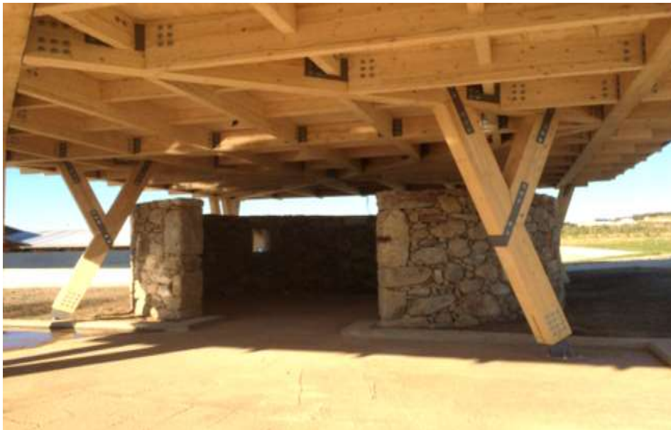
Plate XII: A view of the cafeteria showing local building materials (Source: Matheus, 2019)
