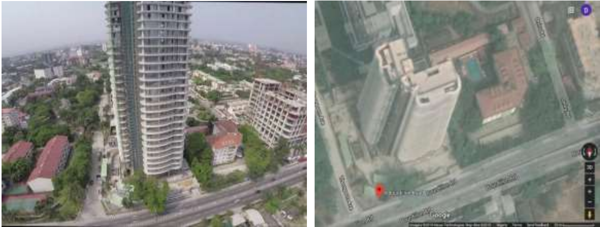
Plate XI: No. 4 Bourdillon's Adjacent Structures and Roads for Easy Communal Transit Source: No. 4 Bourdillon (2019)
