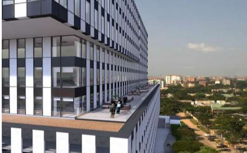
Plate IV: Curtain Walls and Balconies Source: Heritage Place (2019)
