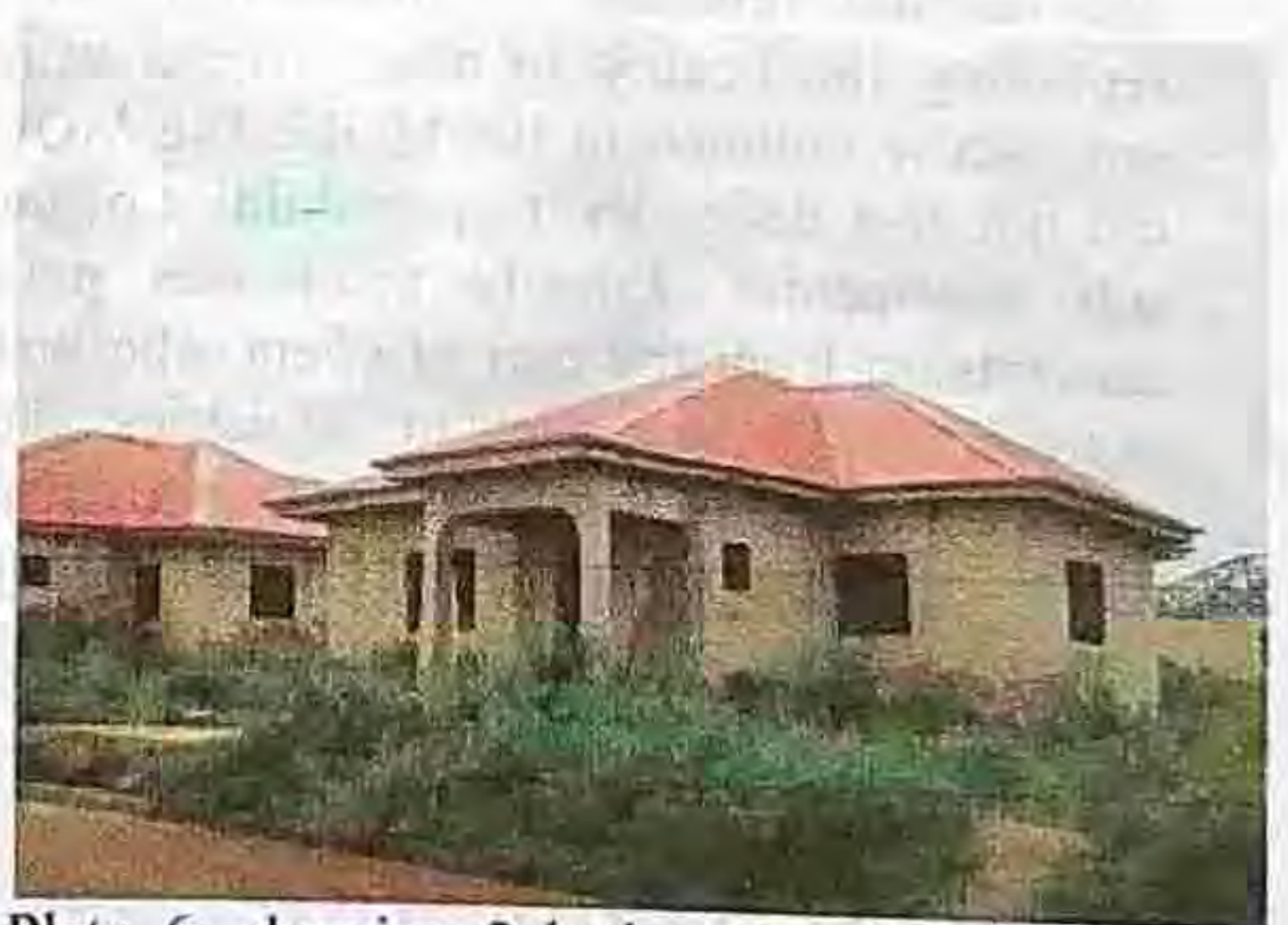
Plate 6: showing 2 bedrooms after repairs were carried out: source authors' field survey 2011
