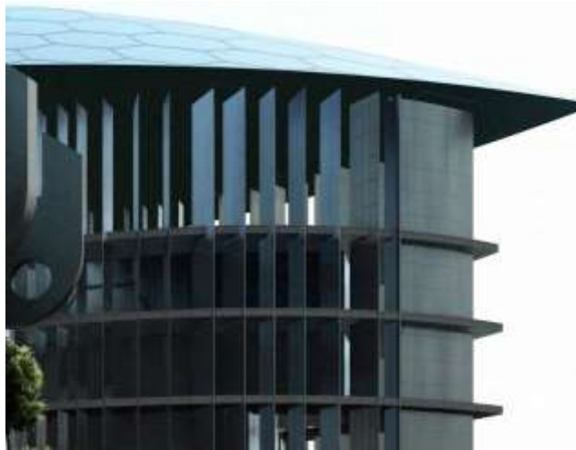
Figure 4.12: 3-Dimensional Section of the Proposed Civic centre Showing the breathing walls and louvers
