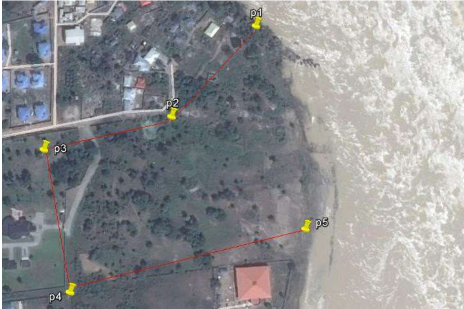
Fig 1.3: Selected Site for the Proposed civic centre at confluence River Lokoja, Kogi State, Nigeria
