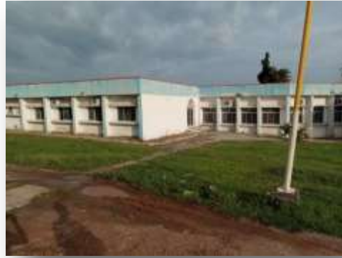
Plate XI. Roof Overhang at Abdulsalam Youth Centre Source: Author's fieldwork (2018)
