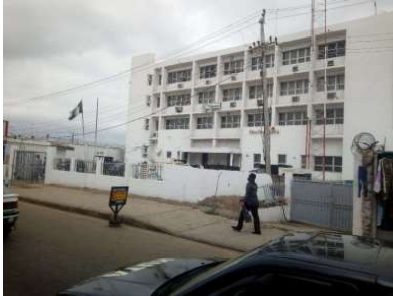
Plate VI: Access gate and perimeter fence at Adekanola house
