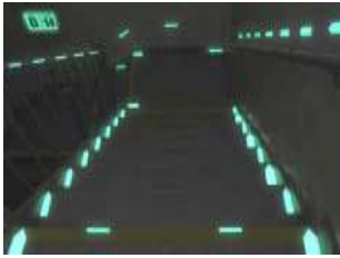
Fig 2.8: Self-illuminating markings on a staircase (Source: Building and Construction Authority, 2005)
