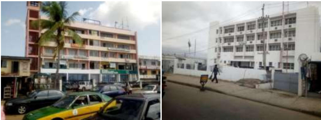
Plate XII: Stand-off distance observed at Aminulshola Plaza in Ilorin. Plate XIII: Stand-off distance observed at Adekanola Building in Ilorin. (Source: Author's fieldwork, 2018)
