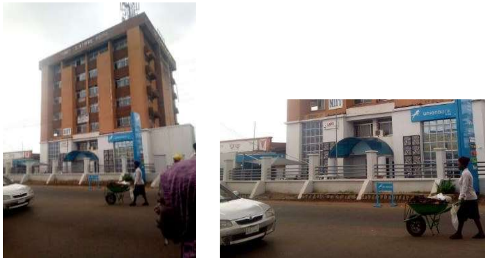
Plate I: A view of TiamiyuOlatinwo house (Source: Author's fieldwork, 2018)
