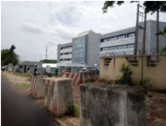
Plate III: Anti-ram walls at Harmony holdings (Source: Author's fieldwork, 2018)
