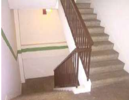
Fig 2.10: Reinforced concrete staircase cores
