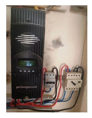
Fig. 10: Photo view of the Charge Controller Assembly
