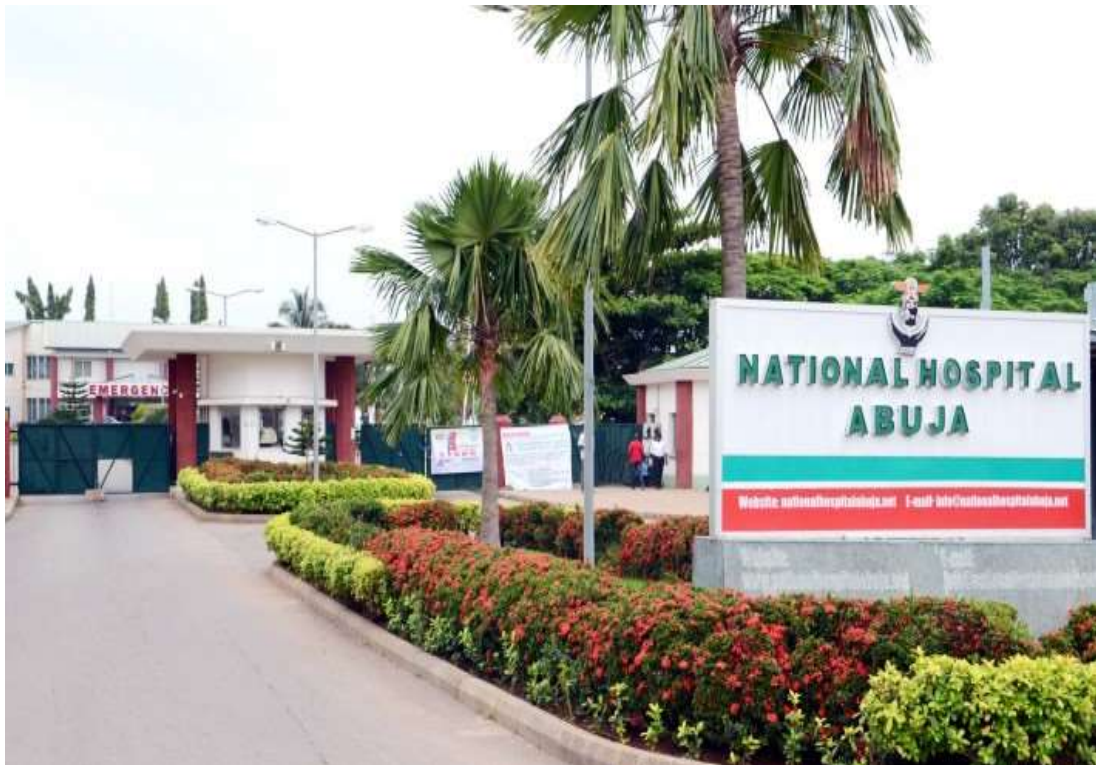
Plate I: Entrance Gate of the National Hospital Abuja (Source: Author's Field Work, 2019)
