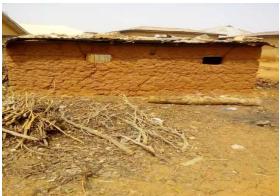
Plate XXV: Size of Windows and the use of Zinc for Roofing (Source: Author's Field Work, 2019)
