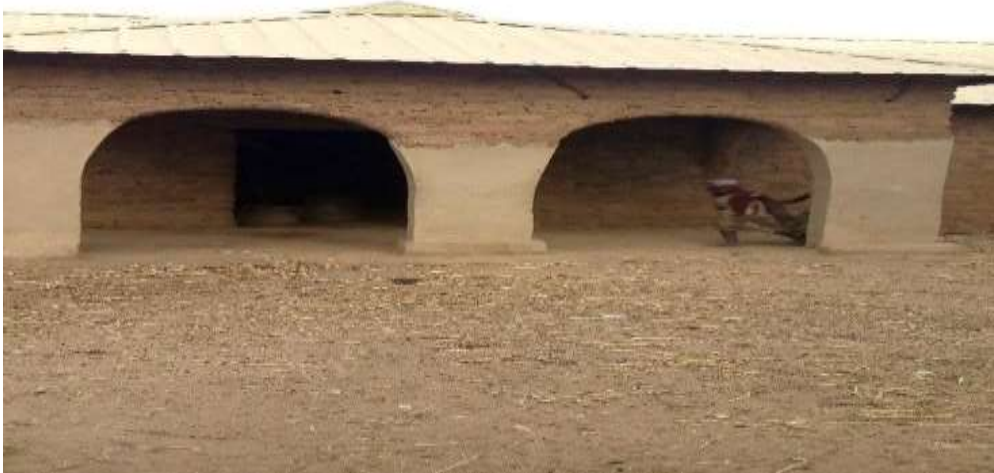
Plate XXXIII: Entrance to the Compound (Source: Author's Field Work, 2019)
