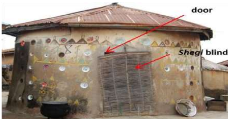
Plate XV: Typical Nupe circular building showing a Door and decorations on the wall (Source: http://www.journalofafricanarts.com (2017))
