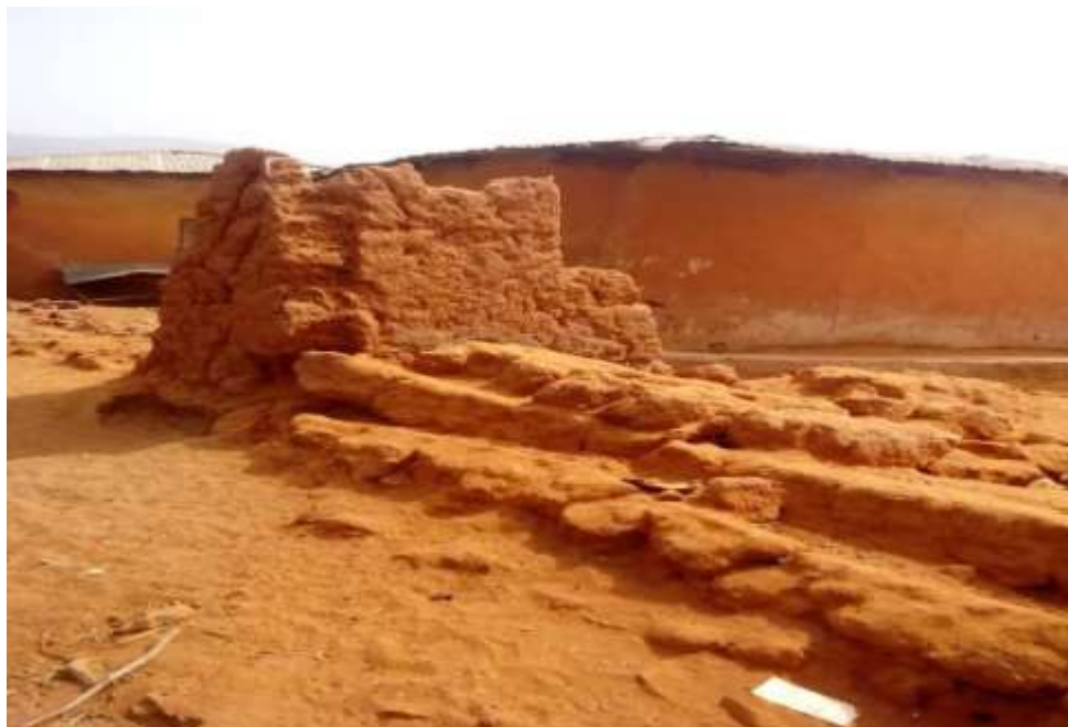
Plate XXIV: Building under Construction in the Compound (Source: Author's Field Work, 2019)
