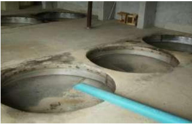
Fig. 6: Underground Firing Evaporation System
